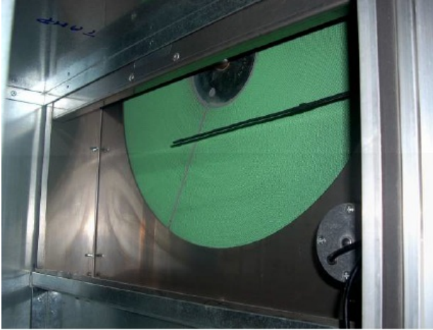
Figure 1: rotary desiccant wheel
