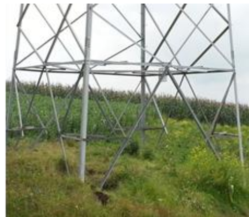
Figure 2. Tower with all its redundant steel members.
