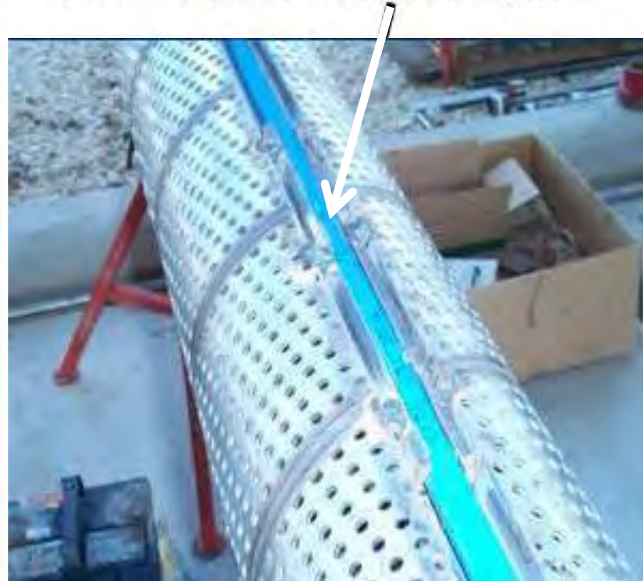
Control line located in sand screen groove
