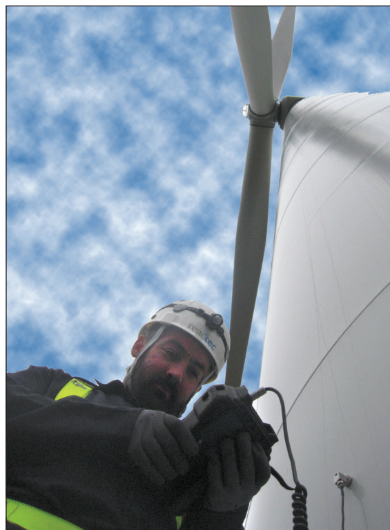
Brett monitoring vibration of a wind turbine tower with a hand held accelerometer.
