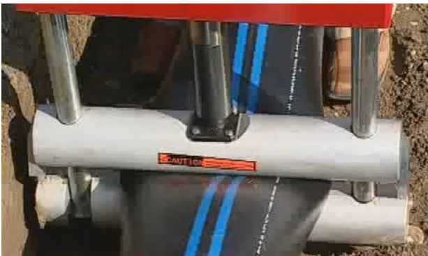
Figure 1: Squeeze-off of PE pipe
