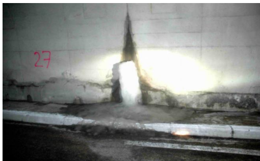
Figure 1. Pack of ice coming from a joint and spreading onto the walkway [7]
