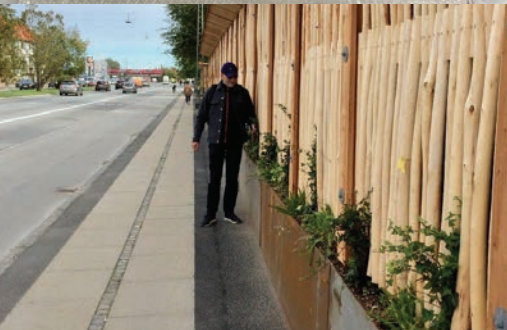
FIGURE 9 An overhead view of the completed structure and a street-side view of the urban green screen.
